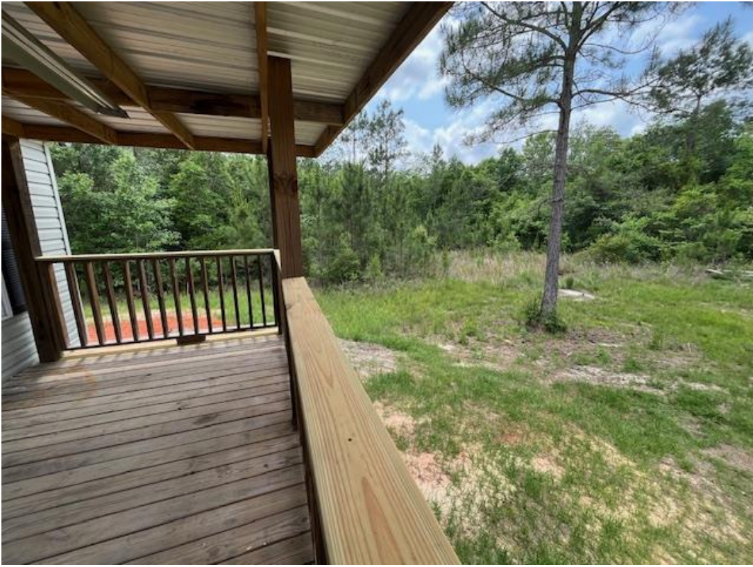
View from covered front porch
