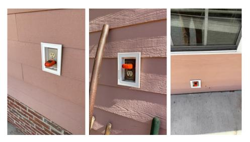
Improve: Up to date and tighter weatherproof covers should be installed on the exterior outlets as noted to prevent moisture intrusion and damage to the wiring.
