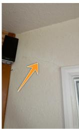
Monitor: Signs of structural settlement were observed at the location(s) noted. If the cracks have not already been repaired, repair cosmetically and monitor for future recurrence.
