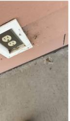
Improve, Safety Issue: The installation of a ground fault circuit interrupter outlet(s) is recommended at the location(s) shown. A ground fault circuit interrupter (GFCI) offers increased protection from shock or electrocution. Up to date weatherproof covers should be installed at all exterior outlets.
