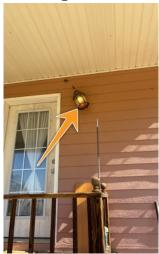
Repair: Loose light fixtures as noted should be tightened and properly mounted to prevent exposure of the wiring and loosening of wiring connections.
