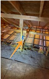
Repair: All open junction boxes as noted should be fitted with cover plates.
