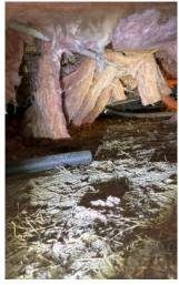
Repair: Insulation was missing or displaced. Adding proper Insulation will increase the efficiency of the home. Have a contractor or qualified handy person reposition and replace insulation where necessary.
