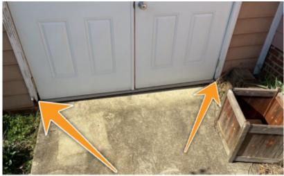
Repair: Damage was noted at the door frame. Consult a carpenter or qualified handy person for further evaluation and repair.
