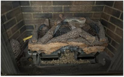
Repair, Safety Issue: The fireplace chimney could use cleaning due to the presence of builtup soot in the chimney from the gas logs. All flues and gas connections should be checked on an annual basis for proper safety.
