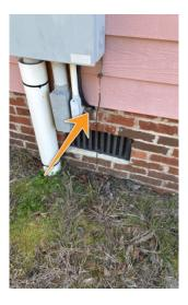
Repair: Penetrations through the veneer for mechanical and electrical components should be sealed with mortar to prevent water, rodent and insect entry. Foam is a poor sealant as it can be chewed through by rodents and deteriorates in the presence of UV rays. Seal around the penetration with silicone caulk or mortar.
