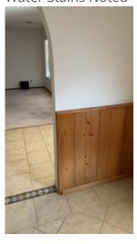
Evaluation, Repair: Water stains were observed at the walls/ceilings in the noted location. Elevated moisture was found in this area. Recommend having a certified contractor evaluate and repair accordingly.
