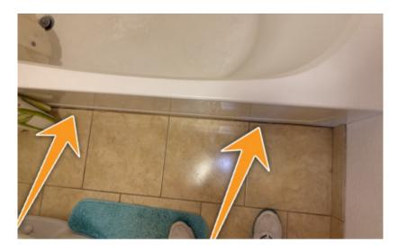
Repair: Cracked, deteriorated, and missing bathtub and/or shower enclosure grout and caulk as noted and should be replaced to prevent moisture intrusion into the wall and floor framing.
