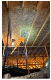
Monitor, Future Repair: Stained and possibly rotted roof decking and/or framing was noted in the attic which appears to have been caused by previous roof leaks. This material should be checked for damaged when re-roofing and replaced as necessary.
