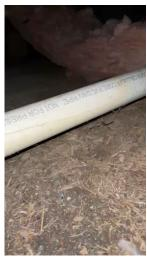
Repair: The waste piping as noted does appear to be smaller than typically found. Small main waste lines can cause potential restrictions. No slow drains were found at the time of the inspection. Recommend having a certified contractor evaluate the waste line size and slope and improve accordingly.
