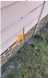
Repair: Loose siding was noted, especially at the location(s) shown, which should be re-nailed and secured to prevent moisture and possible rodent intrusion into the structure. All nail holes, butt joints, and other openings in the siding should be caulked and sealed.
