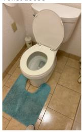
Repair: The toilet at the location noted was loose and needs repair. Have the wax ring checked for leaks and the toilet properly bolted to the floor.
