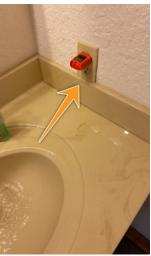
Repair: Loose outlet(s) as noted should be tightened to prevent the loosening of the wiring connections in the future.
