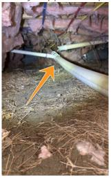
Repair: Some of the water supply piping as noted lacks adequate support (typically required every 2-3 feet). This condition could lead to future leaks at the joints and excessive vibration of the piping. Have a plumber check all piping support in this area and make repairs as necessary.
