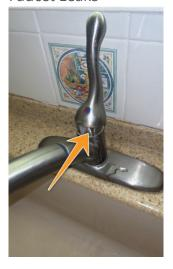
Repair: Some of the faucets leak slightly as noted. This typically indicates that washers inside the handles or valves need replacement.
