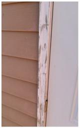
Monitor, Future Repair: The exterior wood trim components will need caulking and painting in the near future to prevent future damage to this material. Any damaged wood should be repaired or replaced as needed. Make sure all holes in the siding and trim are filled and sealed. All utility penetrations (e.g. piping, vents, and light fixtures) should be properly caulked to prevent moisture intrusion.
