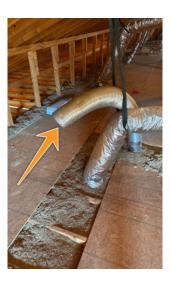
Improve: Bath fans discharging into the attic as noted should instead be vented to the building exterior to limit humidity build-up in the attic.
