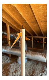
Repair: It appears that a plumbing vent stack is terminating into the attic as noted. This condition could allow sewer gas to collect in this area if the stack is active. A plumber should investigate this condition and either extend the vent through the roof or otherwise have it capped off if not in use.
