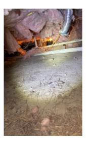
Repair: A moisture barrier should be installed on the crawl space floor to limit humidity build-up in the area, which can promote termite infestations and mildew growth.
