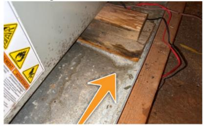
Monitor, Possible Repair: Water staining in the overflow pan was noted. Recommend continuing to monitor for any water buildup in the overflow pan. It is recommended to have all HVAC components evaluated once a year for routine maintenance and cleaning.
