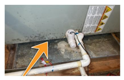
Repair, Safety Issue: Evidence of possible microbial growth and mildew was noted at the furnace at the location pictured, which should be cleaned as needed by an HVAC service company. All ductwork and other components should be checked for further growth and cleaned as needed.
