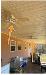
Repair: The ceiling fan did not operate when tested using normal controls. Consult the seller for additional information, or consult an electrician for replacement of the unit.
