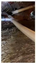
Repair: The drain piping as noted is leaking. A plumber should check all piping and
