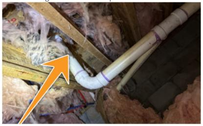
Repair: The floor structure as noted shows evidence of advanced water damage and rotting.
