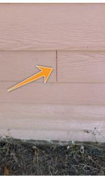
Repair: Gaps and openings in any veneer can allow water penetration into the wall cavity. Properly caulk or grout all gaps in the exterior veneer, paint as needed.
