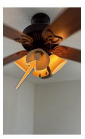
Monitor, Possible Repair: Some of the lights did not come on with the wall switches as noted. First replace the bulb and see it the fixture will operate, if not have an electrician check all lighting fixtures for operable bulbs and then check circuits for proper operation. Consult with the seller concerning all switch locations and/or automatic switches that may be controlling the lights and ceiling fans, if any.
