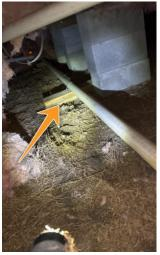
Repair: All wood debris and/or trash should be removed from the crawlspace. Organic debris in the crawlspace increases risk of termite infestations.
